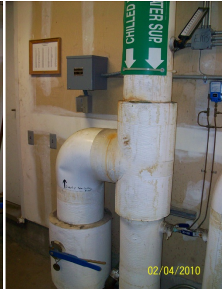
CHILLED WATER CONNECTION FROM CAMPUS CENTRAL PLANT
