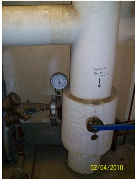
CHILLED WATER CONNECTION FROM CAMPUS CENTRAL PLANT
