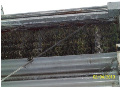
FILL MEDIA CONDITION – EXTENSIVE DAMAGE
