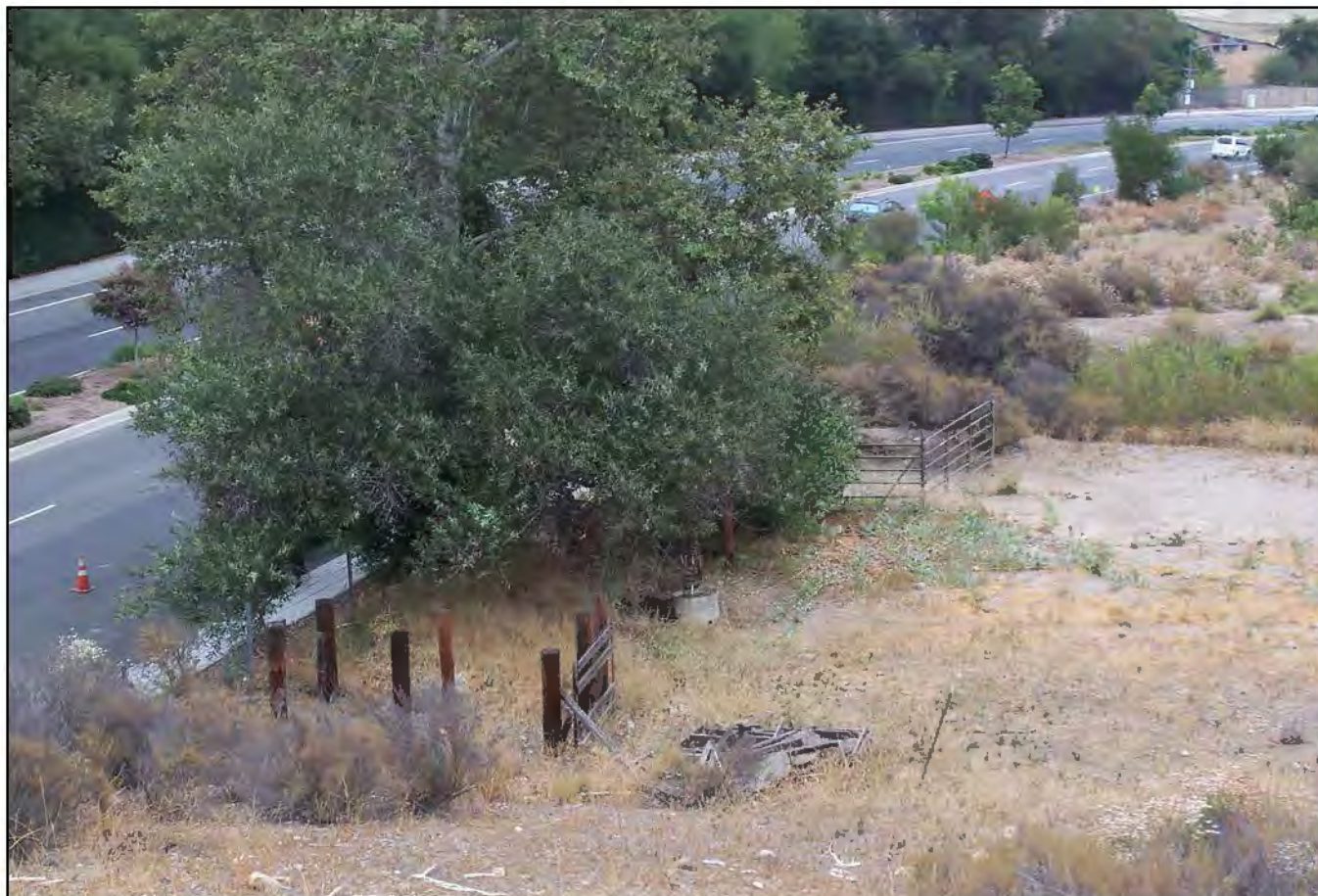
Remnants of the cattle chute and cattle loading corral are in the foreground of this photograph. The water trough is located underneath the willow tree near the center of the photograph, and the cattle gate and dirt access road are situated in the top-right of the photograph (view to the southeast from atop a nearby hill; photograph taken July 16, 2014).
