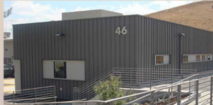
Emergency Ops Center
